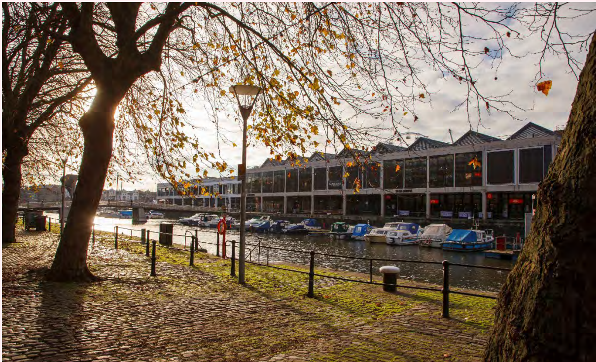
The long, low-slung profile of the transit sheds emphasises the defining horizontals of the Listed dock walls, the surface plane of the water, and the length of St Augustine's Reach. 84 degree field of view from Narrow Quay
